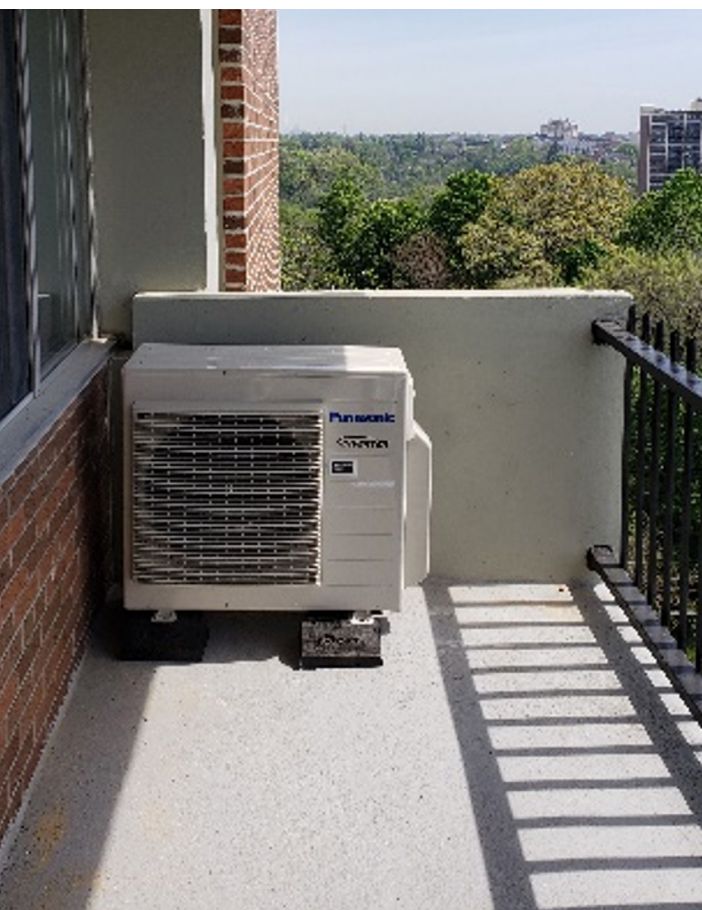
Outdoor Unit installed on balcony
