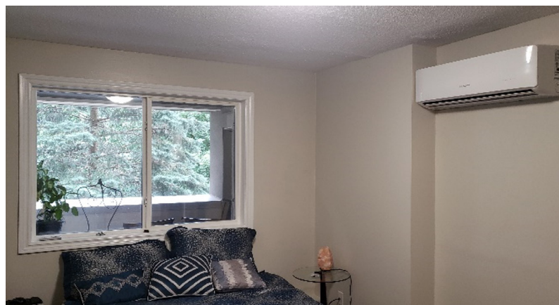
Indoor Unit installed in bedroom
