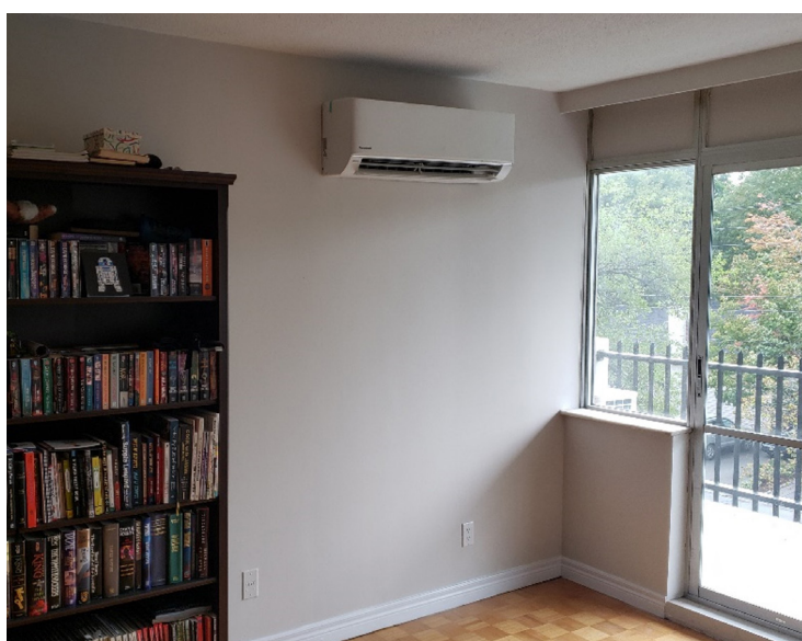
Indoor Unit installed in living room
